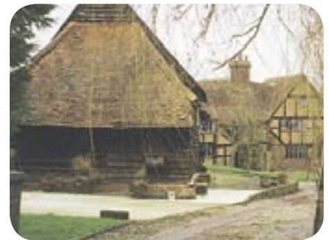
Carpenters Farmhouse, Goddards Lane
