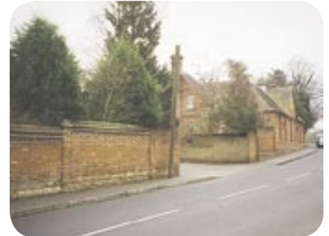
The former coach house and brick boundary walls to The Old Rectory
