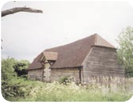
Breach Farm Barn
